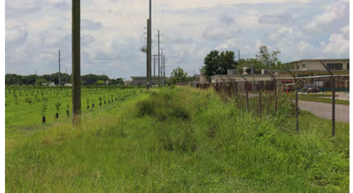
4. The power line easement could be repurposed with the addition of a sidewalk that connects Maple Street to Story Road.
