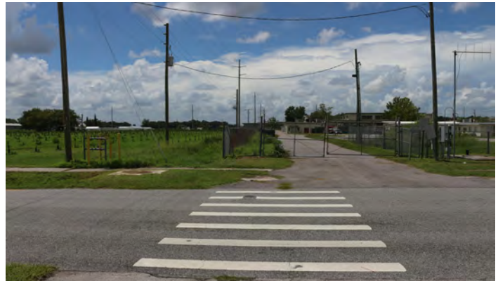
3. The sidewalk disappears next to the vocational school.
