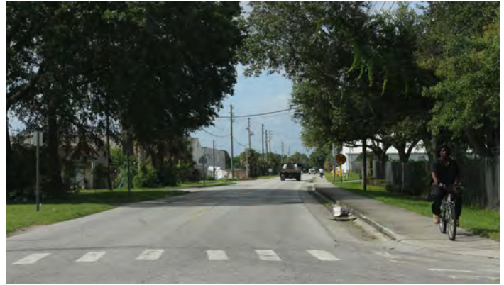
Existing Conditions on 9 th Street
