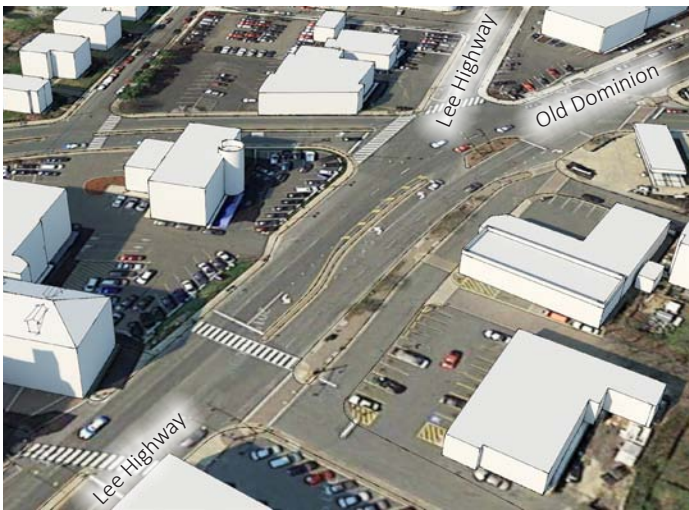
above: Existing conditions, Cherrydale and the 5-points intersection, aerial view.
